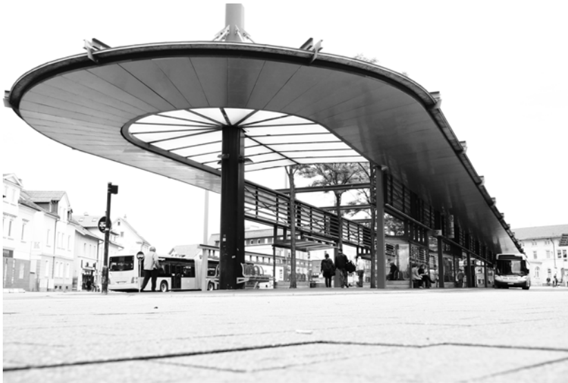
Jens-Fabian Thönnissen: Busbahnhof Aalen Bus station, Aalen Gare routière à Aalen Stazione delle autolinee a Aalen
